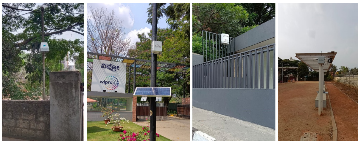
Figure 2: Examples of sensor node installations for ambient air quality monitoring following the United States Environmental Protection Agency (US EPA) guidelines, ensuring free airflow (no large walls or trees nearby).
