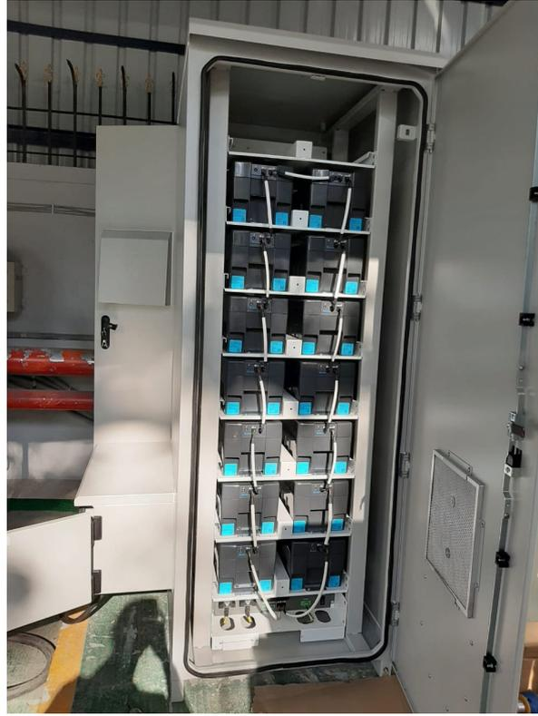
Figure 6: Snapshot of the (internal) battery bank showing 14 battery modules in series. The total energy capacity of the bank is 43.5 kWh.
