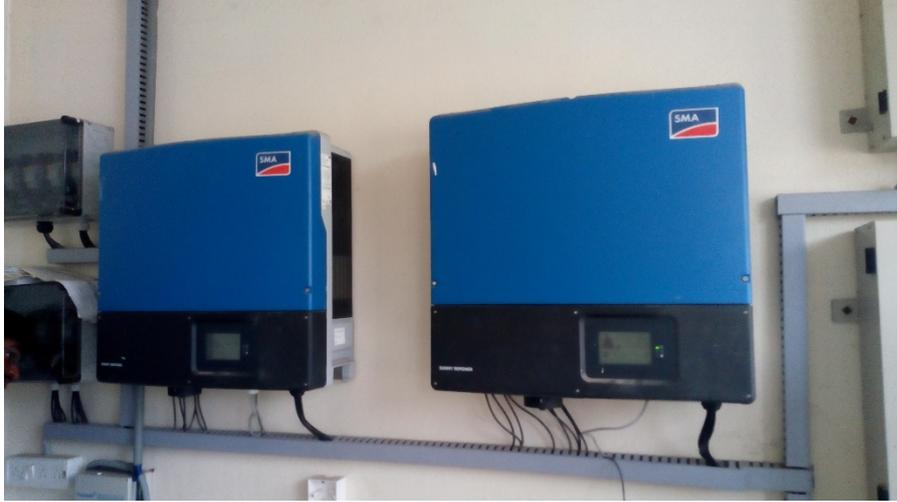
Figure 4: Existing string inverters of capacity 20 and 25 kW, connected to the 40 kWp RTPV system
