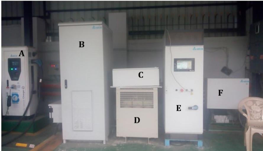
(A: Bharat DC 001 charger, B: lithium-ion battery bank, C: MPPT block, D: transformer, E: PCS, and F: distribution box)
