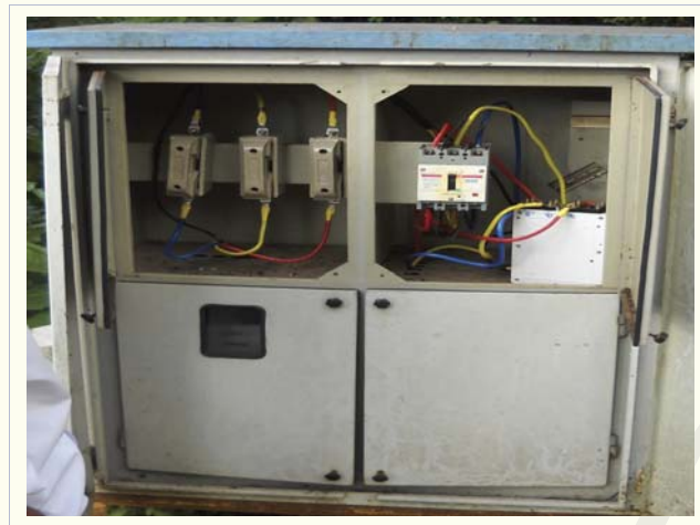
Street Light Control System
