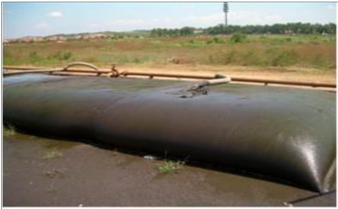
**Figure 20: Schematic View of Geobags in Malaysia**
