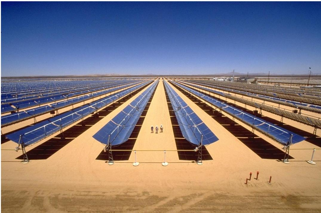
**Figure 2.1: Parabolic trough collectors**
