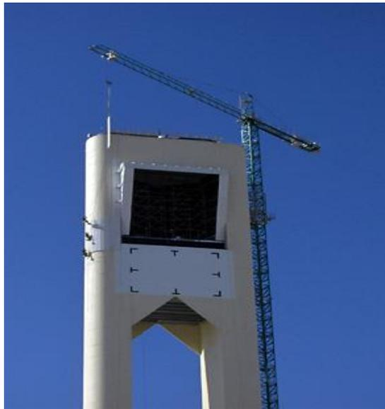
**Figure 2.5: Cavity receiver used in PS-10**
