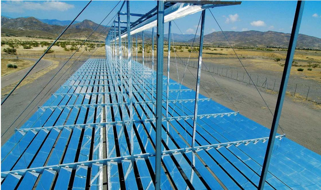
**Figure 2.13: Linear Fresnel Reflector system**
