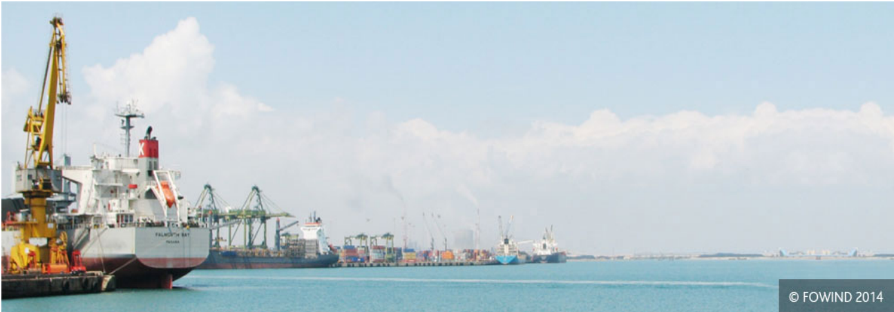
Vessels harboured at the South Breakwater in VOC port, Tuticorin
