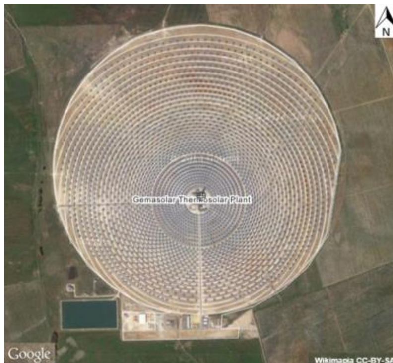
Figure 3: Gemasolar ST Plant in Spain
