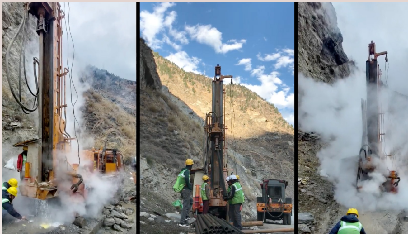
Figure 3.9: Geothermal drilling in Himachal Pradesh. Source: Geotropy.
