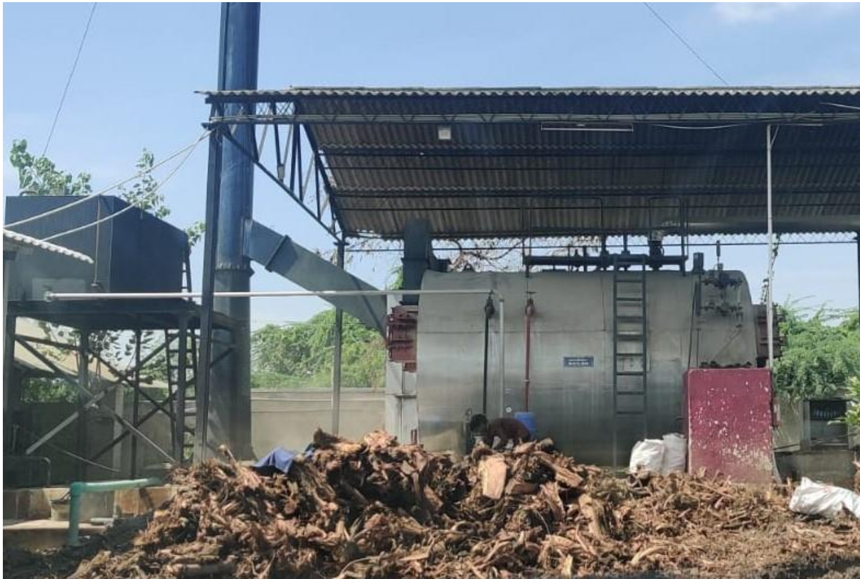
Image A1. Wood-fired boiler for which an energy audit was performed during a field visit in Tiruppur
