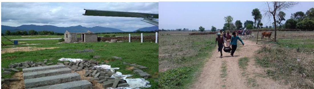
Construction work took off with the support of villagers
