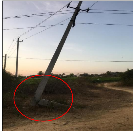
Figure 19: Broken pole
