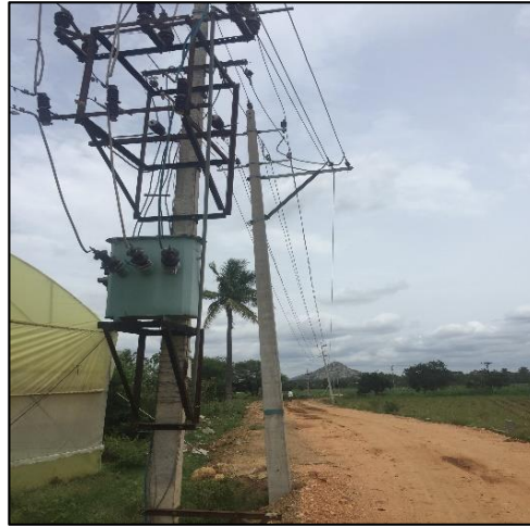
Figure 6: DT without meter (2)
