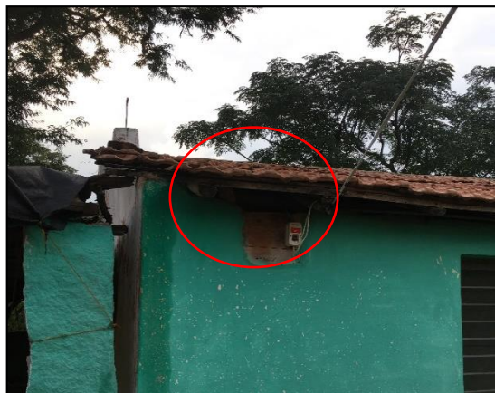
Figure 22: Installation with direct connection (without meter)
