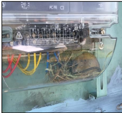
Figure 16: Rat inside the meter
