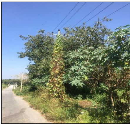
Figure 13: Poles covered with bushes
