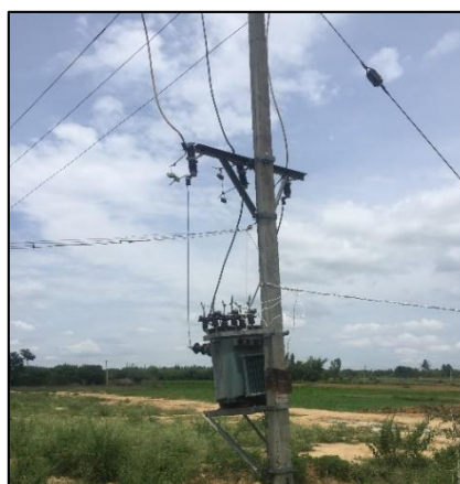
Figure 5: DT without meter (1)
