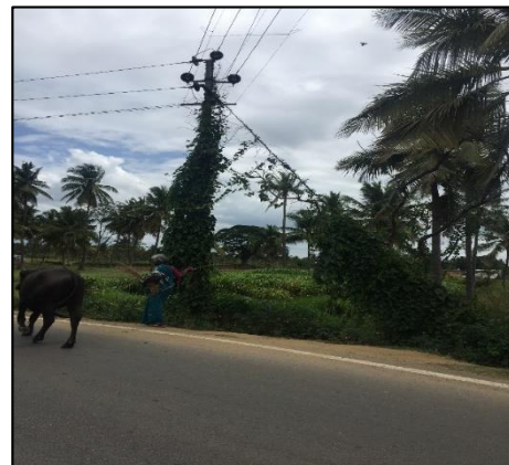
Figure 13: Poles covered with bushes
