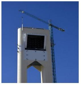
Figure 2.5: Cavity receiver used in PS-10
