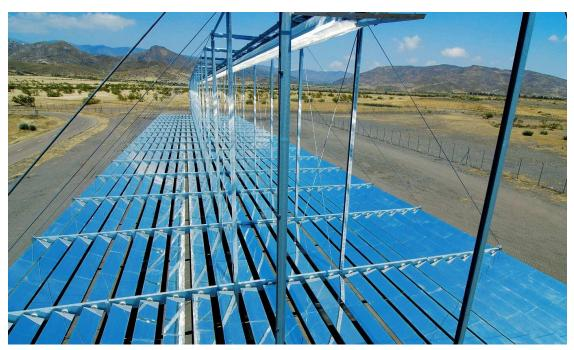
Figure 2.13: Linear Fresnel Reflector system
