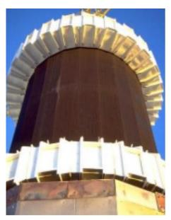
Figure 2.4: External cylindrical receiver used in Solar Two
