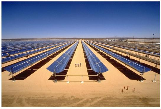
Figure 2.1: Parabolic trough collectors
